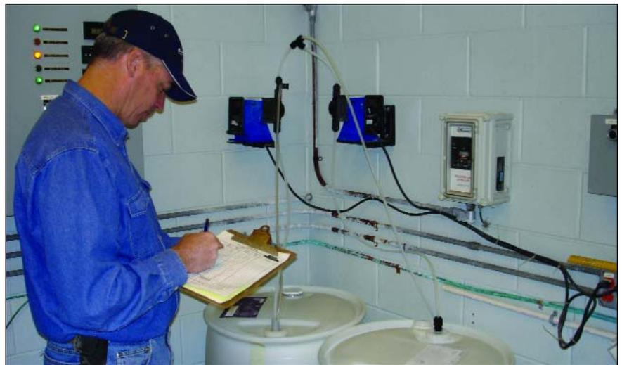
*Paul Strathman, Manager/Operator of Nemaha RWD 3, checks the amount of phosphate pumped during the prior 24-hour period. The RWD presently produces an average of 600,000 gallons per day. With iron content of 0.6 and manganese at 0.13, Strathman says that patrons would not tolerate the staining that might be prevalent were the RWD to not use a good sequestering agent.*
