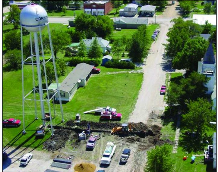
*Volunteers at Corning are shown installing the last section of pipeline, connecting the water storage tank to the main which was installed earlier in the project. The above photo was taken by KRWA Tech Pete Koenig who was instrumental as both inspector and worker.*
