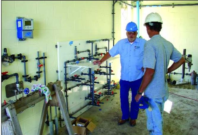
*In anticipation of upcoming regulation changes, the city is installing new chemical feed equipment in order to disinfect with chloramines. Gary Kincy and one of the installers discuss the progress of the project.*
