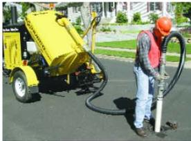
**Valve & Vac:** With this option, clean and vacuum valve boxes prior to exercising. A one-unit operation that can be easily towed to job sites with light duty vehicles.
