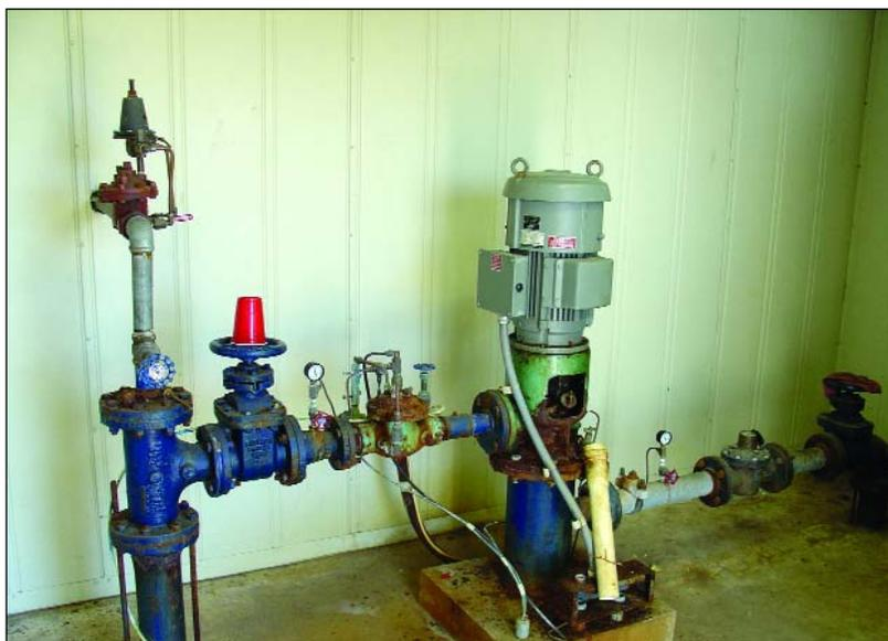
*A booster pump station should have a by-pass or a second pump to allow water flow to continue during times when maintenance is being performed or in case of a pump failure. If the single pump is out of service, there is often no way for the system to maintain water supply beyond the pumping station. Typically, a sanitary survey would identify this sort of deficiency.*
