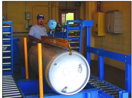
Mike Dommick, Leavenworth Water Department, moves a one-ton chlorine cylinder into place to be loaded into the utility's new ChlorTainer containment systems.
