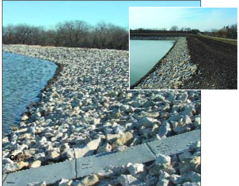
*These photos at Waterville show a rebuilt dike and complete riprap in place to control erosion.*
