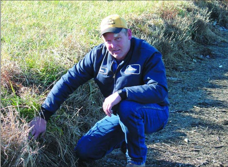
*Dean Hermes, Operator at City of Olpe, shows dike erosion on one of the city's lagoons. The most severe erosion is generally on the windward slopes of the dikes. Most systems are unaware of the extent of erosion until the lagoon level is lowered.*
