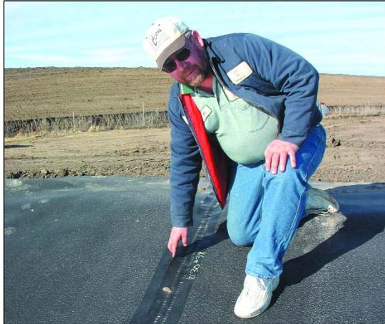
*Jim Knight, Wastewater Operator for the City of Seneca, inspects the lap seam of this vinyl type liner installed on two new wastewater ponds (cells) constructed last fall. Liners such as this are an alternative to riprap to prevent dike erosion, in addition to providing seepage control from the cells which is otherwise typically accomplished by adding clay to the base.*
