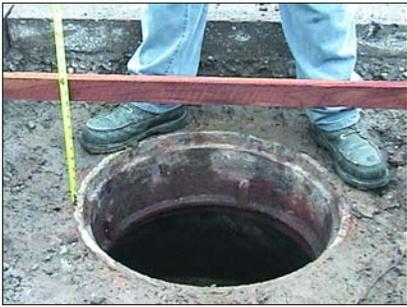
*This manhole needed to be elevated by nearly 2 feet to bring it back to grade level.*
