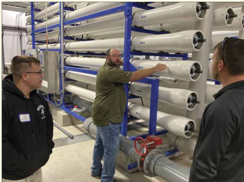
Stuart Leak with Avista Technologies explains how reverse osmosis works to Dylan Chavez with WaterWise Enterprises (L) and Levi Brewer from the City of Haysville (R) during the Reverse Osmosis Treatment System Basics training session held at the Arkansas City Water Treatment Plant on October 17. The Water Treatment Plant hosted multiple training sessions during the month of October.
