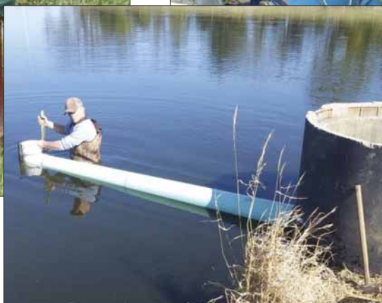
Jason Soloman, Wastewater Tech, installing a new outfall structure.
