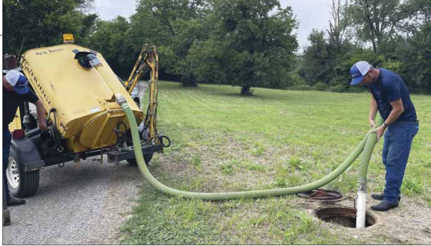
This photo shows one of the two Hurco vac units KRWA operates to help water and wastewater systems clean valve risers and other confined spaces. The unit can also pot hole to help locate buried lines, etc.
