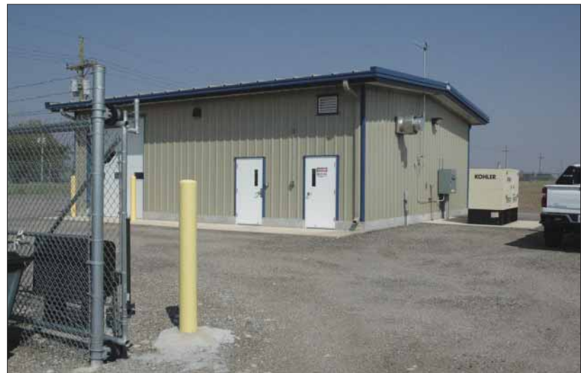
This is the metal pump station building with standby generator and chain link security fence.
