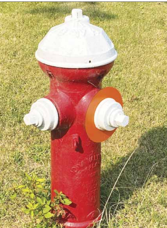
Orange ring under cap indicating a flow of 500 to 999 GPM.
