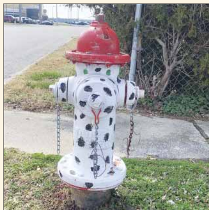
Painted puppy dog hydrant with Red top indicating less than 500 GPM flow.
