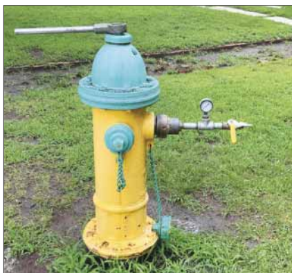
Pressure testing fire hydrant with bleed valve.
