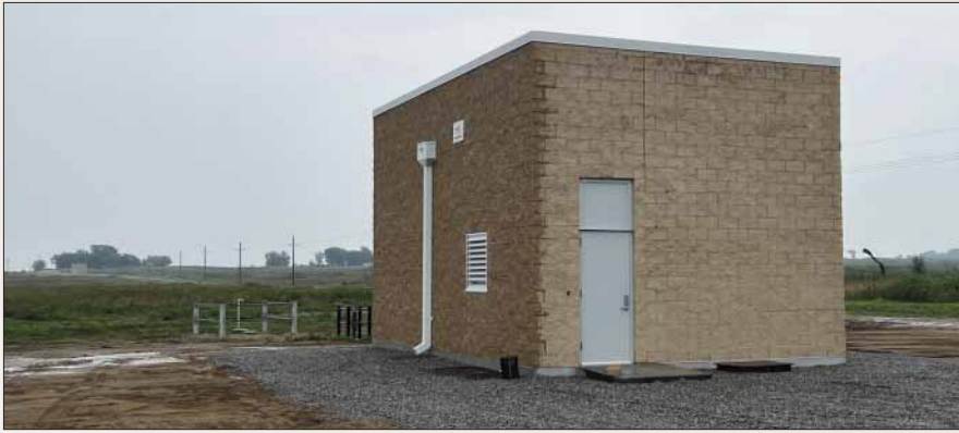
Wellhouse No. 15 is ready for pumping equipment to be installed. Wellhouse No. 16 is visible approximately ⅓-mile to the east, on the left side of the photo. Well No. 17 is behind the hill further east.
