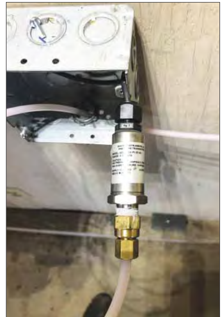
A pressure transducer, often called a pressure transmitter, is an electromechanical device designed to measure pressure with a high degree of accuracy. Pressure transducers sense applied pressure and output an electrical signal by using a combination of mechanical and electrical components. The most common transducer outputs are voltage and milliamps.
