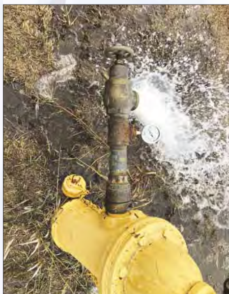
A pressure relief valve should be installed on a distribution system even if other control options are being used. It’s a safety valve in case of some other failure.
