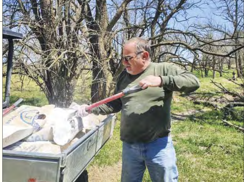
KRWA Wastewater Tech Charlie Schwindamann spreads lime over the bypassed sewage in the creek.
