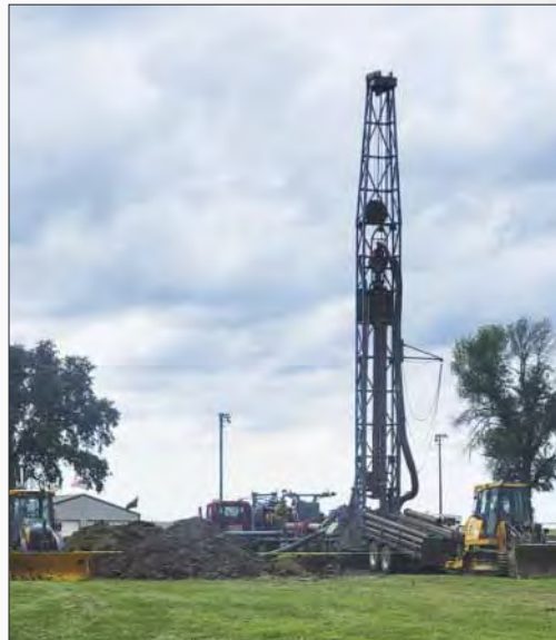
This photo shows drilling rig operated by Sargent Drilling.
