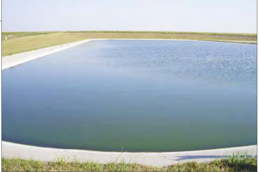
This photo shows an example of a well-maintained lagoon cell. If possible, grass should be mowed before any inspection or kept at a respectable height at all times. Trees, cattails, and other aquatic plants are well-controlled and not a problem.
