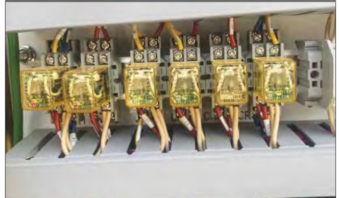
Liquid Control Relay controls the level of liquid in a vessel so that submerged pumps do not run dry.
