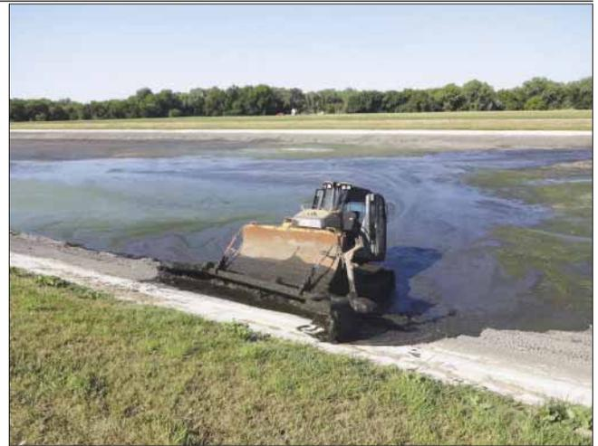
**This is the small bulldozer with a modified blade that was used to collect the sludge slurry and move it toward a pump for ultimate removal. During the day as the sludge started to dry in Cell 1A, wastewater would be pumped from Cell 1B over to Cell 1A to keep the sludge in liquid form so it could be pumped.**
