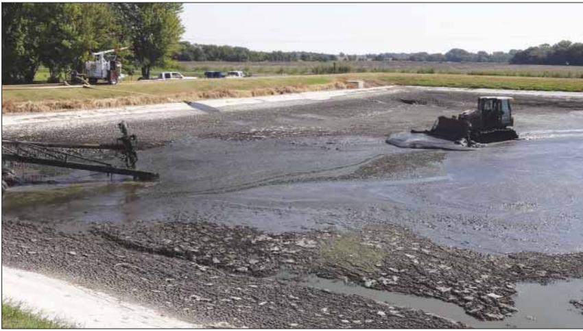
**This small bulldozer pushes the sludge slurry to a corner to be pumped to the application site. This must be done over and over to get as much sludge as possible to the pump for removal.**
