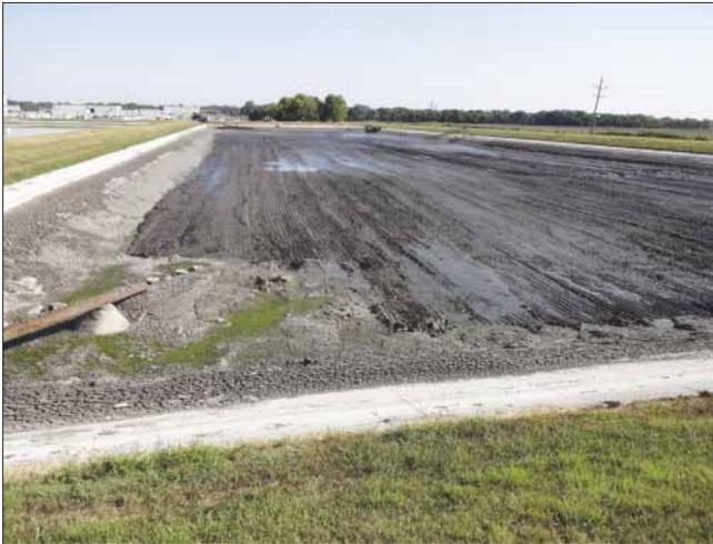
**This photo shows Cell 1A after some sludge was removed. Notice the build-up of sludge in the corner around the influent pipe.**
