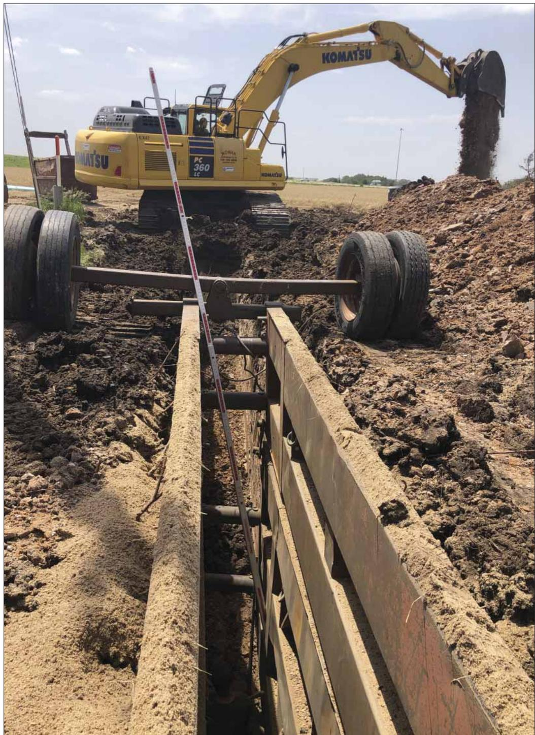
Nowak Construction, Goddard, Kansas begins installation of a new 8-inch sewer line. Because of the depth, this excavation is being caged for safety of workers.
