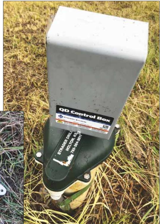
This photo shows a wellhead that is equipped with a pitless adapter.
