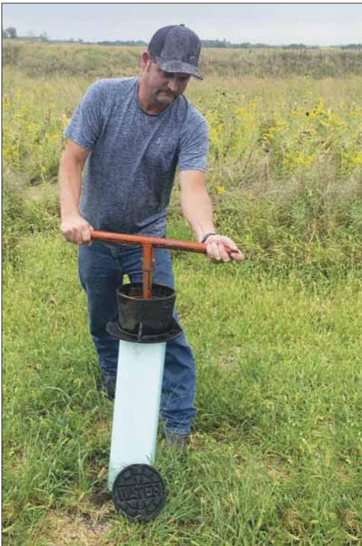
KRWA Tech Tony Kimmi exercises a valve during a water loss survey on a rural system in northeast Kansas. Notice the tilt of the valve riser. This is due to a lack of adequate compaction around the riser or it was not straight and centered at the time of installation.
