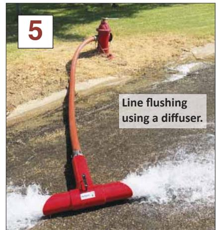
5 Line flushing using a diffuser.
