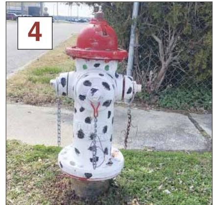
4 Painted puppy dog hydrant with Red top indicating less than 500 GPM flow.
