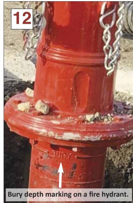
Bury depth marking on a fire hydrant.
