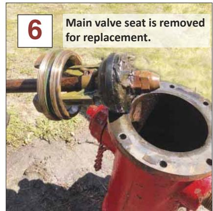
6 Main valve seat is removed for replacement.
