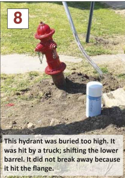
This hydrant was buried too high. It was hit by a truck; shifting the lower barrel. It did not break away because it hit the flange.
