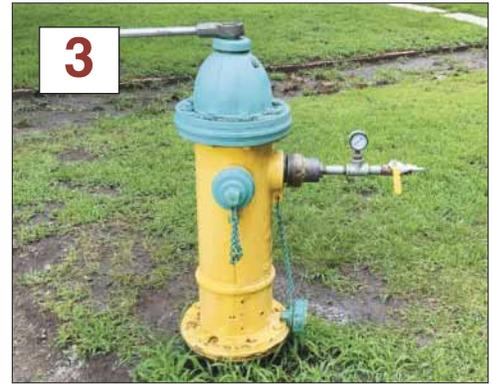
3 Pressure testing fire hydrant with bleed valve.
