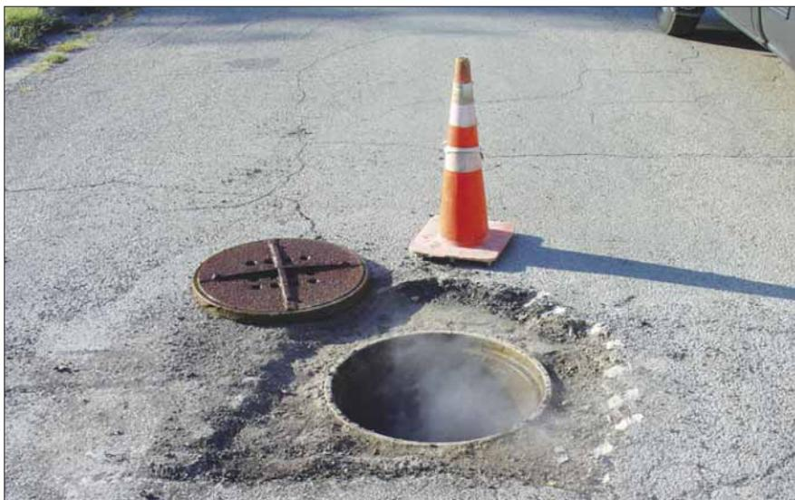
**This manhole was located and excavated to allow for smoke testing of the collection system. This manhole was at least four inches below grade. If access is needed in an emergency due to a sewer backup, it could cost the system thousands of dollars for cleanup because of slow response and having to locate and excavate the manhole.**
