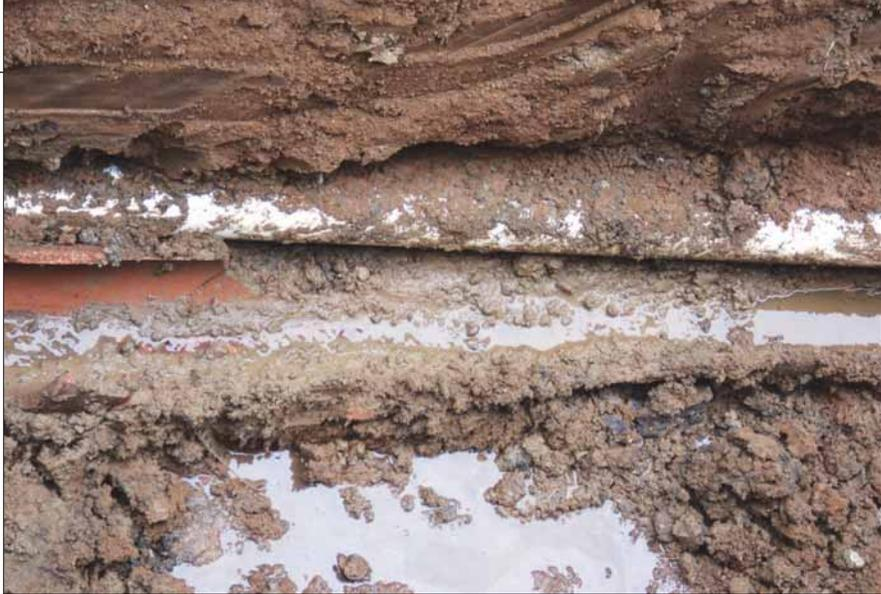
**This photo shows a fiber optic line which has been drilled through a clay tile of a city's collection system.**
