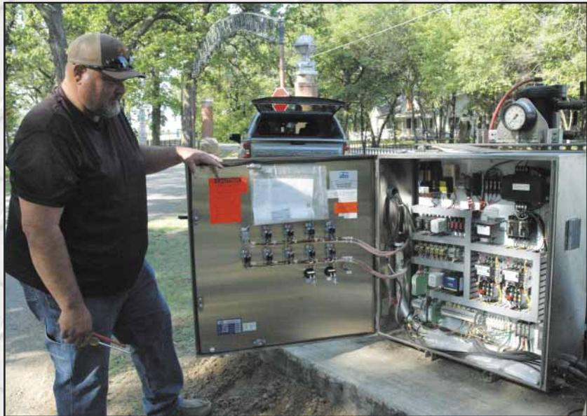
**KRWA Wastewater Tech Brian Bowles conducts a visual inspection of controls on a lift station controls, looking for dark areas on relays and motor starters. Below, he tightens those that were loose.**
