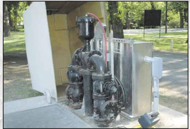
**A wastewater lift station is a pumping station that moves wastewater from a lower elevation to a higher elevation. The benefit of using a lift station in a sewage collection system is that it saves a substantial amount of money in excavation costs.**
