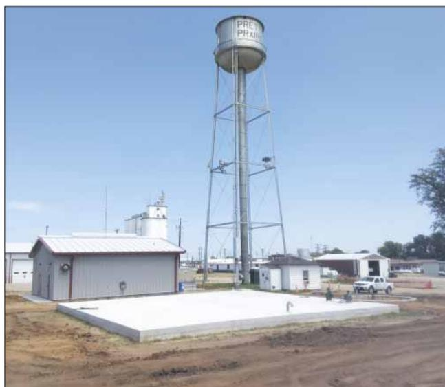
This photo shows the completed clearwell with the two submersible pumps in the lower right corner. The old 50,000-gallon elevated tank in the background was removed later.
