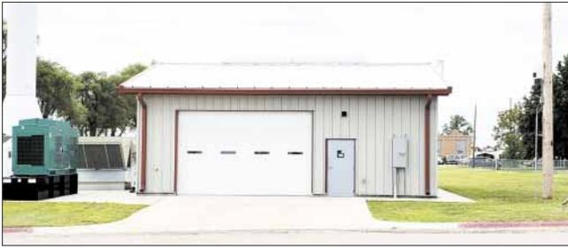
The new treatment plant building houses the RO membranes and a standby generator.
