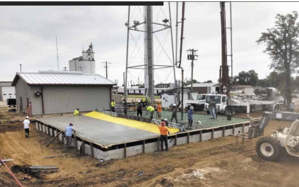
This photo shows the new 150,000-gallon clearwell under construction.
