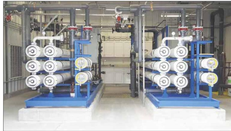
Shown here are the two Pentair RO skids. The skids are operated individually, alternating every 24 hours.
