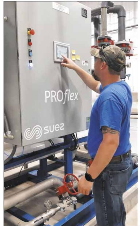
Dustin Jesseph, Water Operator, points to the Human Machine Interface (HMI) touch screen on the control panel. Comm-Tronix, Wichita, Kan, installed the system controls.
