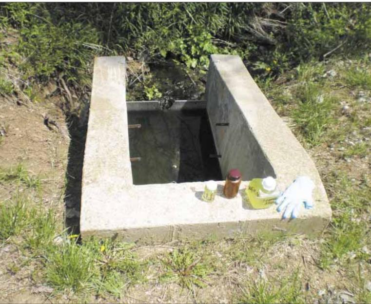
**This is a typical outfall structure for discharge from sewage treatment plant. The best location to collect effluent samples is from flow going over V-notch weir cut into metal stop plate. Also note sample containers used for collecting samples to be analyzed for BOD, TSS, ammonia and *E. coli*.**
