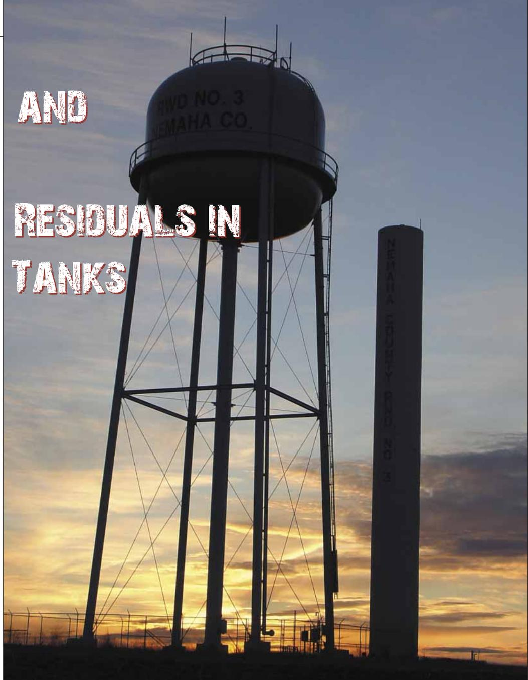
Many rural water districts and cities have increased storage tank capacity as shown in this photo taken in Nemaha RWD 3 where a new 500,000-gallon tank replaced a 12 x 110 standpipe. While not the case in this district, many cities and RWDs have tank capacity beyond what can be effectively utilized without causing concerns for freezing in winter and loss of water quality during summer and fall months.
