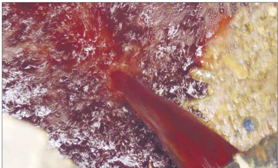
**This photo shows blood from a locker plant entering the city's lift station. While the photo indicates the blood is diluted by other flow, high BOD of more than 100,000 mg/l is not uncommon for whole blood from locker plants.**
