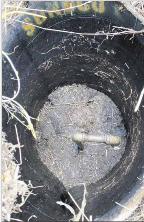
**Some installations of air releases are clearly contamination hazards. This unit is installed in pit, that although covered, allows surface water to enter. Note the lines of debris on the sidewall of the pit, well above the top of the air release vent pipe.**
