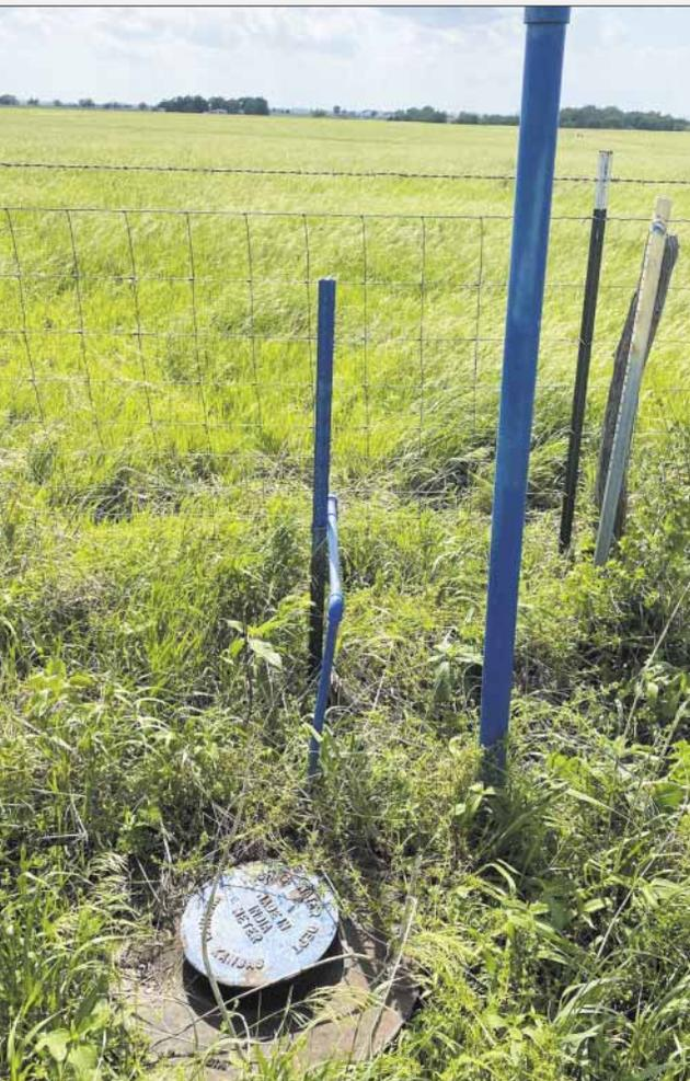
This photo shows a typical valve arrangement and the vent pipe from an air release valve in a rural water system in southeast Kansas.
