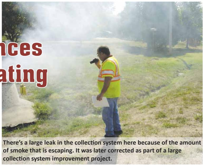
There's a large leak in the collection system here because of the amount of smoke that is escaping. It was later corrected as part of a large collection system improvement project.
