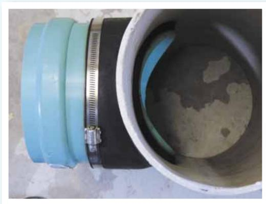
This photo shows one of many types of taps that are utilized by wastewater systems to provide a watertight, secure seal to the sewer main.
