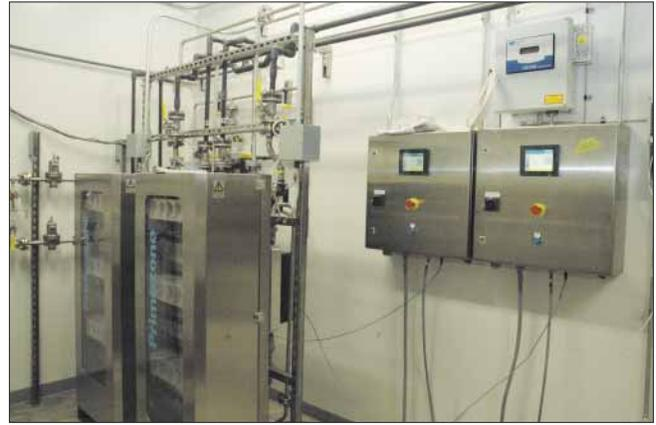
These photos show the oxygen tanks and the Primozone ozone generator that will allow the city to comply with the EPA standard for THMs of 80 ppm.
