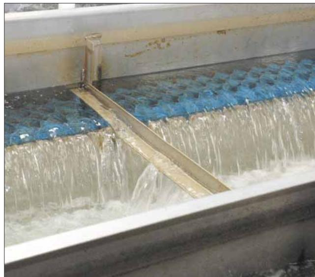
This photo shows the filter being backwashed. Baffled wash troughs are provided in both filters to prevent media loss during the washing process.
