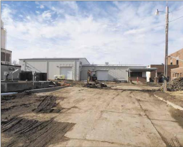
This is a view of the new water plant building containing the two package plants along with the ozone generator, high service and backwash pumps, and an office. The old power plant building that still contains the clearwell can be seen on the right side of the photo. The contractor is still on site to finish cleanup.
