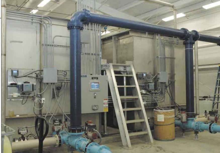
The complete surface water treatment process is contained in these tanks; they replaced the original upflow clarifiers and gravity sand filters.
