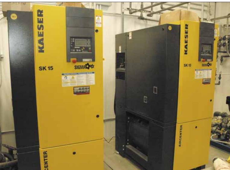
Shown here are the compressors used to produce oxygen for the production of ozone. Ozone is replacing free chlorine as the primary disinfection procedure.
