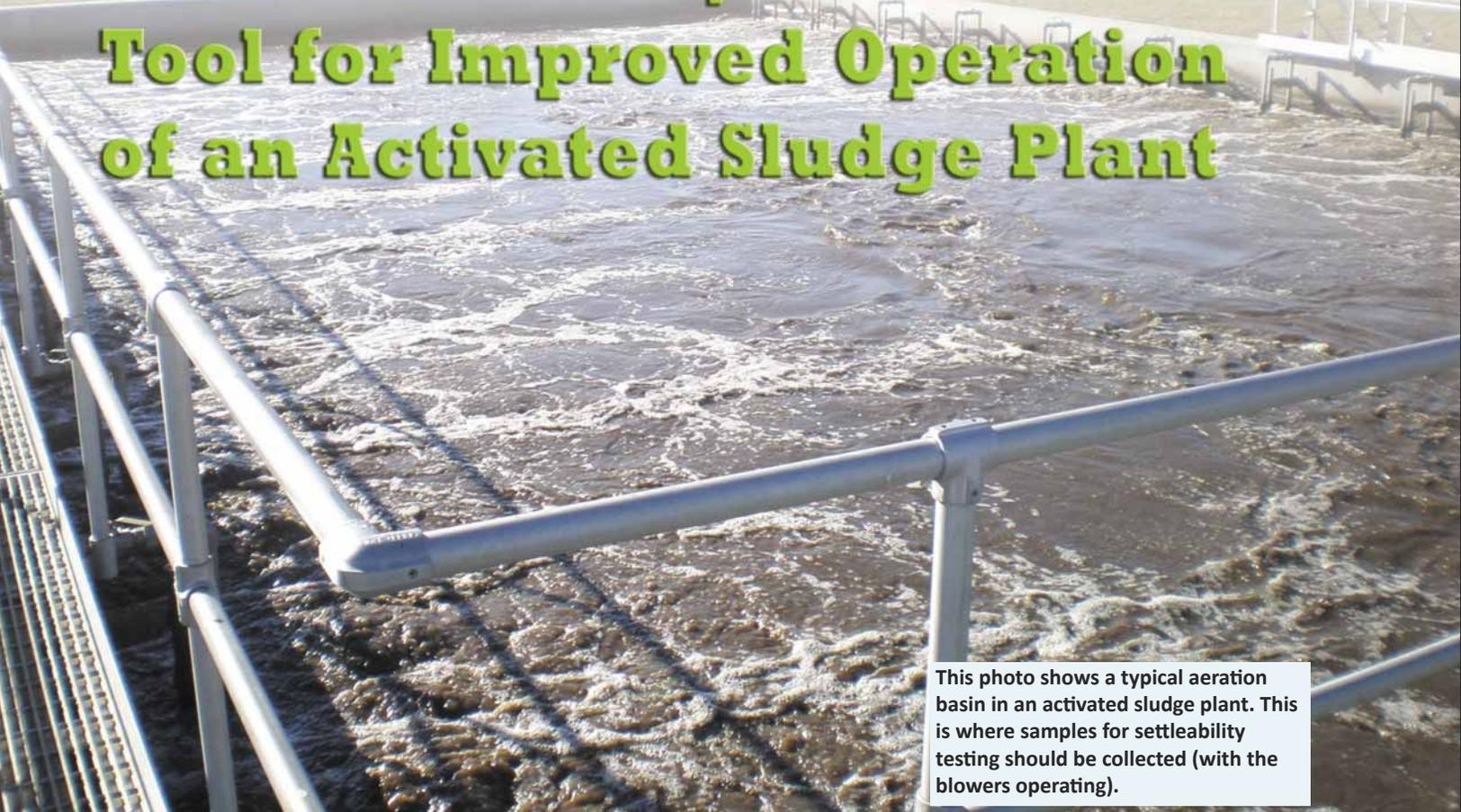
This photo shows a typical aeration basin in an activated sludge plant. This is where samples for settleability testing should be collected (with the blowers operating).
