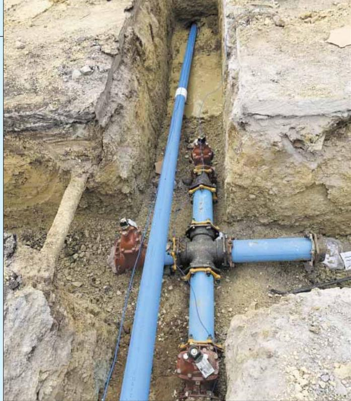
Bore being pulled in, and valve cluster at an intersection.
