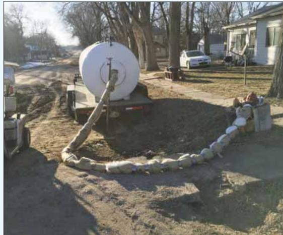
**KRWA provided assistance to the city of Republic by setting up one of the Association's potable pressure tanks. Insulation was added to help prevent freezing of connecting piping.**
