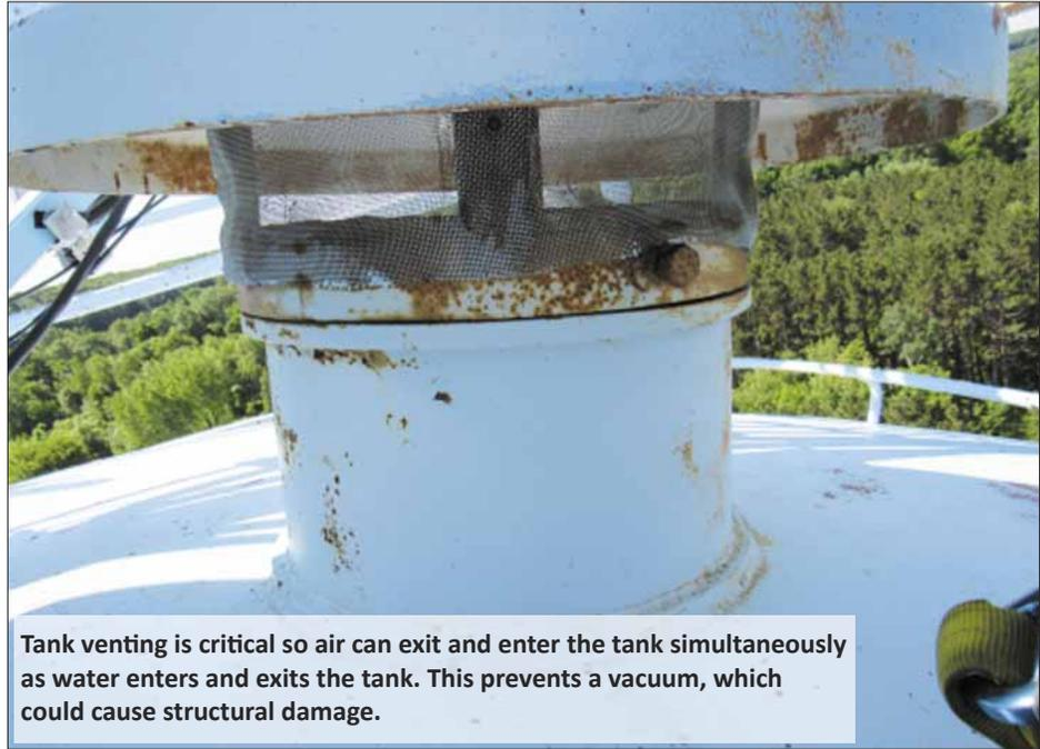
**Tank venting is critical so air can exit and enter the tank simultaneously as water enters and exits the tank. This prevents a vacuum, which could cause structural damage.**
