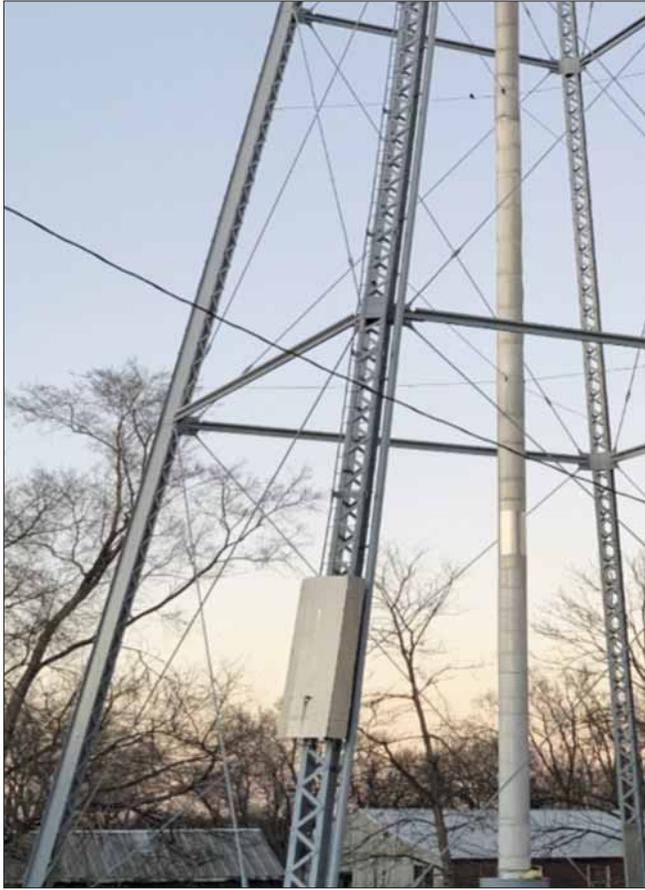
Since 2001, water storage facilities have been designated as federally-protected site. Access should be restricted through multiple layers of protection such as the ladder guard shown in this photo.
