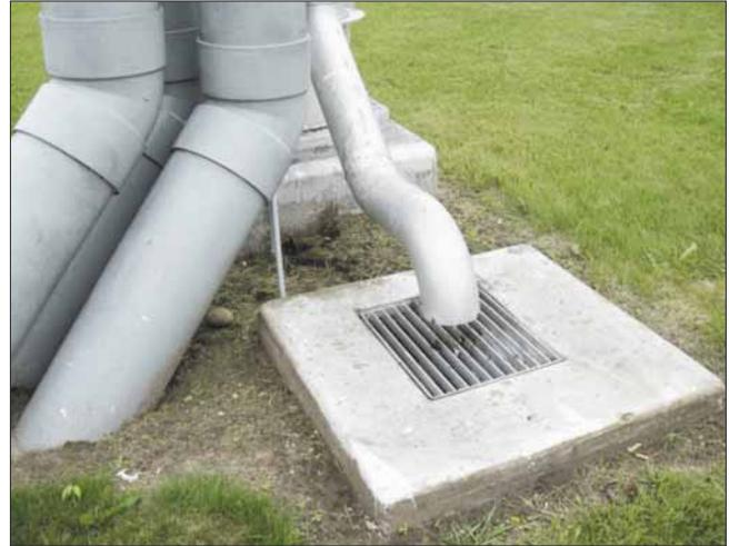
Tank overflow pipes need to be adequately screened and should have adequate relief of the overflow pipe within 12 to 24 inches or an air-break above the ground.
