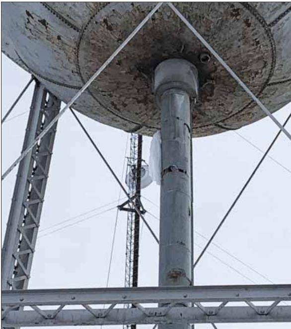
The stem pipe at Republic broke just below the bowl of the tank. Note the four-foot chunk of ice on the pipe.
