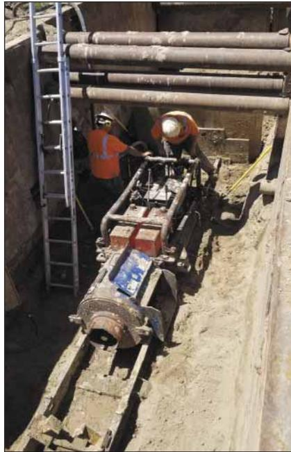
A subcontractor on the project is setting up to bore Highway 83 to install a 12-inch casing for a 6-inch main.
