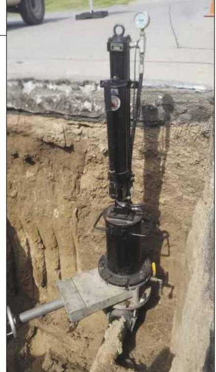
A Hydrastop is being done to allow replacement of a valve that was broken in the off position while the city was doing a shut down so the contractor could compete a tie-in.
