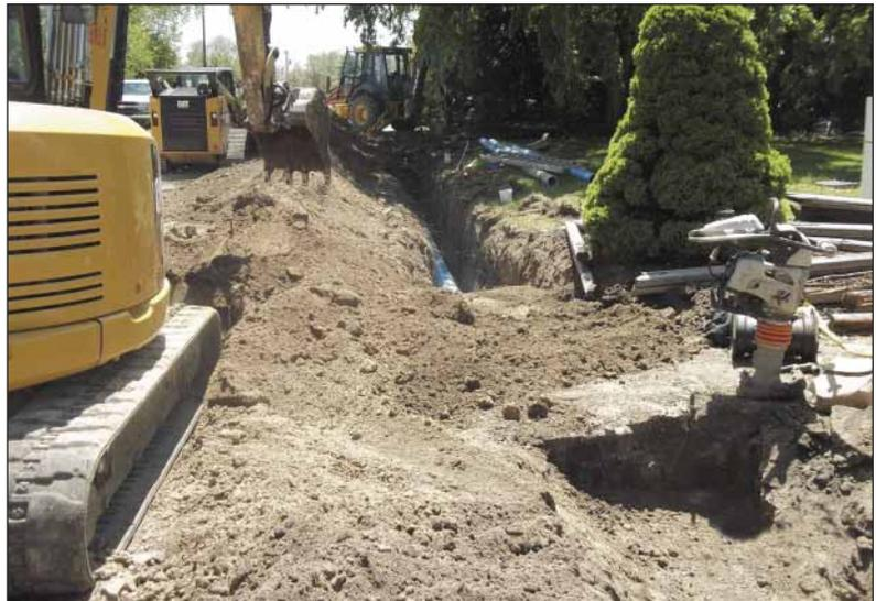
This photo shows new PVC water line being installed in a very busy area.
