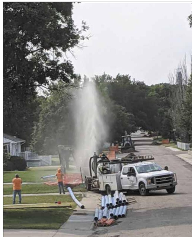
Oh shucks! The geyser shown in this photo occurred when the contractor caught a service line while pulling pipe back and caused a corp stop to break off the old main. The city was in the process of shutting down line valves when the water finally caused an opening forming a geyser.
