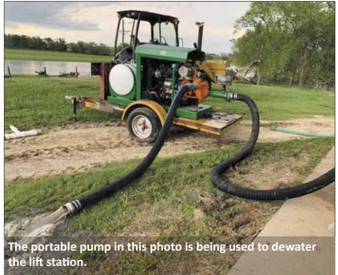
The portable pump in this photo is being used to dewater the lift station.
