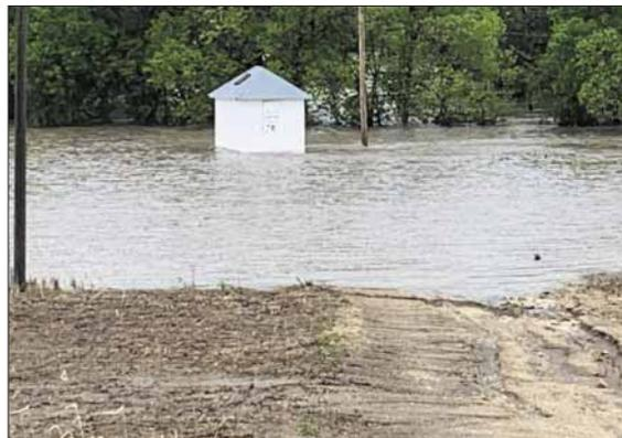
**Note the flood water level at Well No. 6. This well was to have been built above the flood plain but it has been flooded on at least one previous occasion.**
