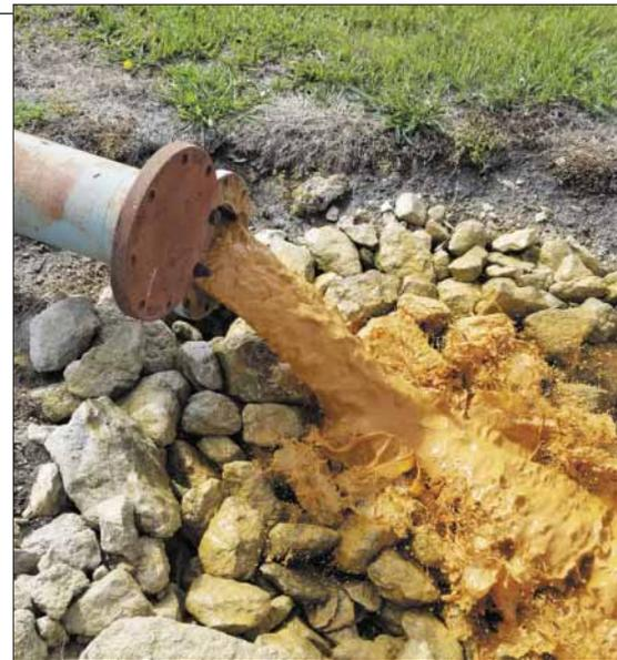
These two photos show water running clear, then not so clear – are the results of a line pigging procedure. The clear water was 12 minutes into the pigging event and the murky water was after 25 minutes. This water system routinely pigs the line from the well field to the water plant on a quarterly basis.
