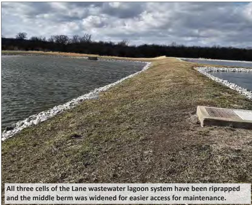
**All three cells of the Lane wastewater lagoon system have been riprapped and the middle berm was widened for easier access for maintenance.**
