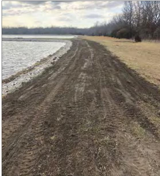
Soil was hauled in to finish the inside of the berm to a 3:1 slope as outlined in KDHE’s minimum design criteria.
