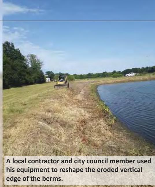
A local contractor and city council member used his equipment to reshape the eroded vertical edge of the berms.
