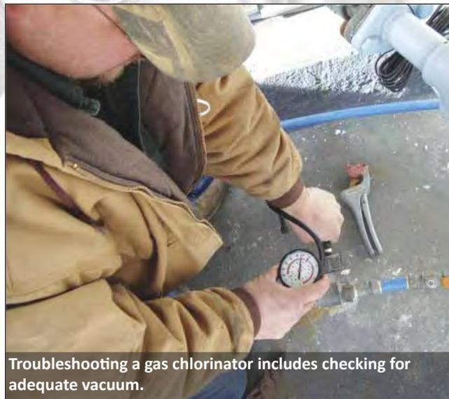
Troubleshooting a gas chlorinator includes checking for adequate vacuum.
