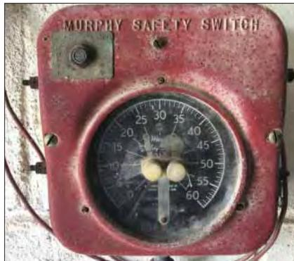
Before today's automation, many water system storage tanks were controlled with the aid of a mercrod type mechanical switch such as this Murphy Safety Switch, Model 6045.
