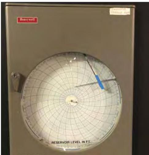
Before today's automation, many water system storage tanks were controlled with the aid of equipment such as this Honeywell level indicator (chart recorder). This unit was installed in the 1990's and remains in service today.
