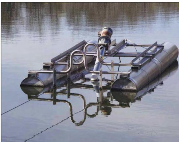
This photo shows one of the three, two-horsepower aerators on Cell 2 of the city of Leocompton’s wastewater lagoon.
