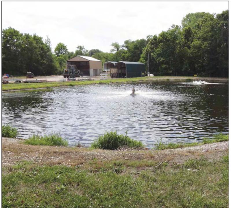
The 0.9-acre primary cell (Cell 1) of Lecompton's lagoon is equipped with two, five horsepower surface aerators to keep dissolved oxygen at satisfactory levels. This cell had four feet of sludge on the bottom that was eventually removed and land-applied.
