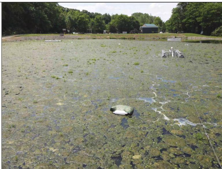
**This photo shows Cell 2 completely covered with filamentous algae mats. These mats block sunlight which is needed by algae to produce oxygen needed by bacteria to break down organic matter. Such a situation can adversely affect treatment and effluent quality. The mesh bag with float in the foreground is barley straw introduced to control the algae.**
