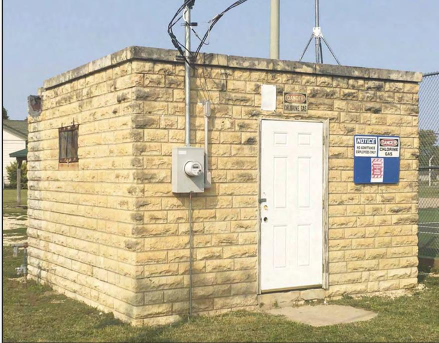
This wellhouse is approximately one city block from the center of the EF3 tornado that hit Chapman just after 10:00 p.m. on June 11, 2008. The limestone structure was able to withstand the strong wind with minimal damage.
