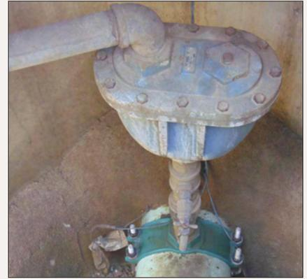
**This photo shows an air relief valve made of cast iron installed on a public water system main.**
