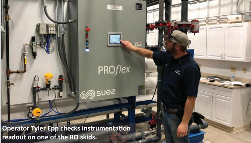
Operator Tyler Epp checks instrumentation readout on one of the RO skids.
