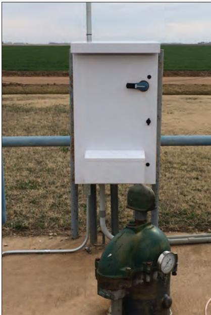
The city's well is now equipped with a variable frequency drive.
