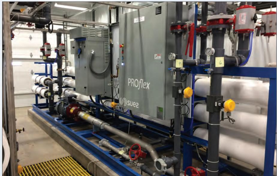
The plant is equipped with two PROflex RO skids by Suez Water Technology. A new 50,000-gallon tank was also included in the project.
