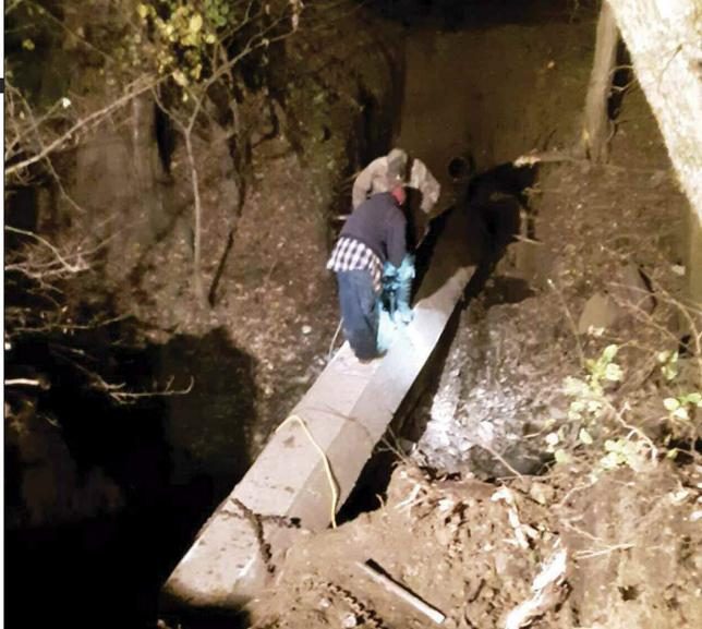
When the city of Toronto's main sewage line to the treatment plant ruptured in a creek crossing, city staff and KRWA staff worked through the night to temporarily repair the line to keep sewage from flowing into Toronto Reservoir.
