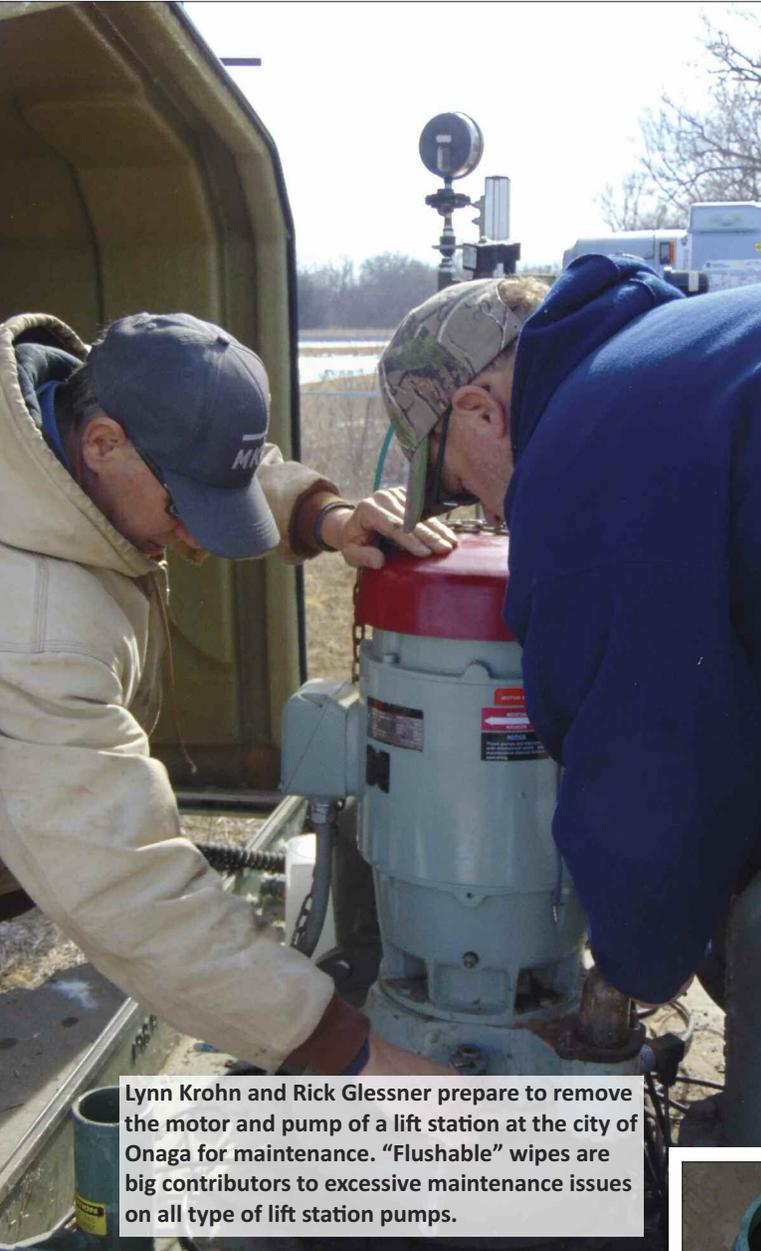
Lynn Krohn and Rick Glessner prepare to remove the motor and pump of a lift station at the city of Onaga for maintenance. “Flushable” wipes are big contributors to excessive maintenance issues on all type of lift station pumps.
