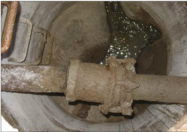
The sewer main shown in this manhole was discovered many years ago as part of a water system replacement project. The water main was relocated to the edge of the street to meet the required minimum horizontal separation distance of ten feet.
