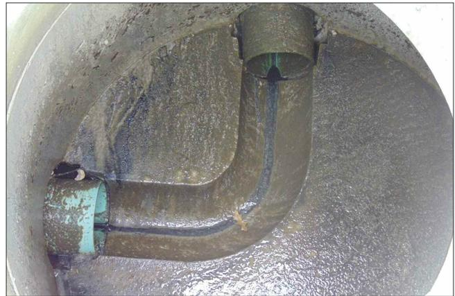
This photo shows the need to have manholes at all changes of direction to allow for cleaning and repairs.
