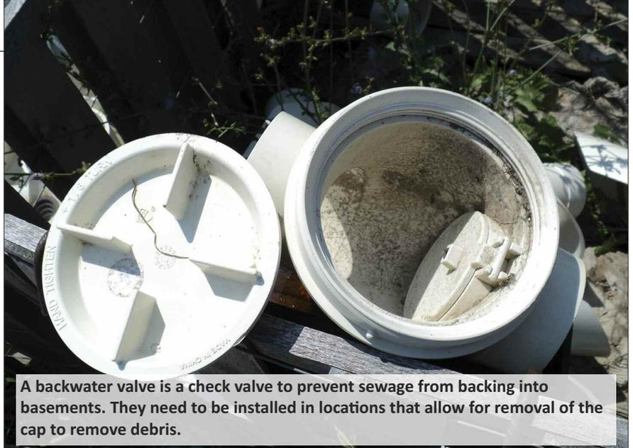
**A backwater valve is a check valve to prevent sewage from backing into basements. They need to be installed in locations that allow for removal of the cap to remove debris.**
