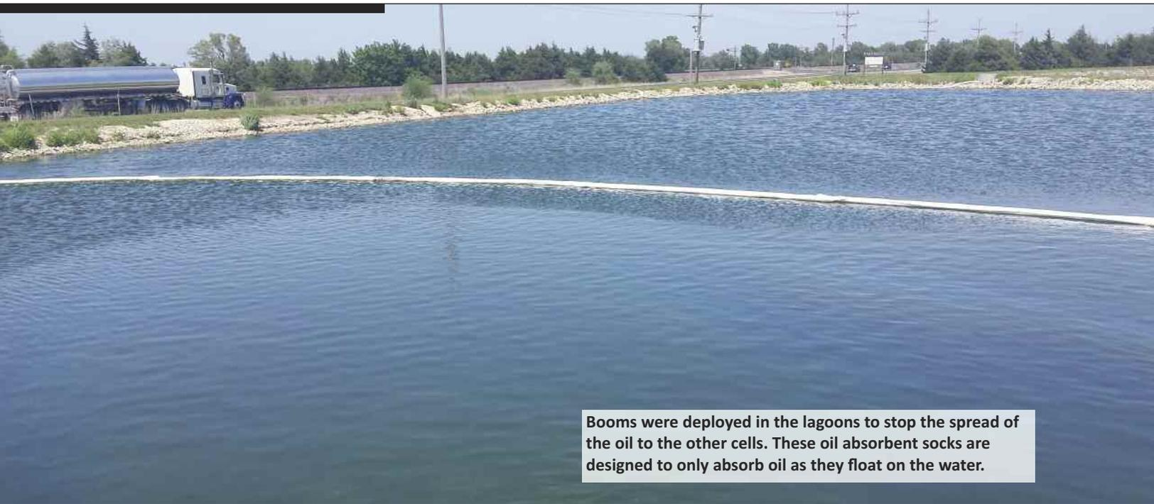
**Booms were deployed in the lagoons to stop the spread of the oil to the other cells. These oil absorbent socks are designed to only absorb oil as they float on the water.**
